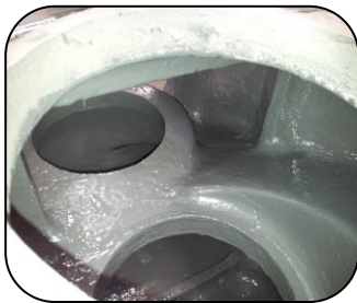
Sea water filter operating at 95°C coated with 205 Ceramic HT Fluid
