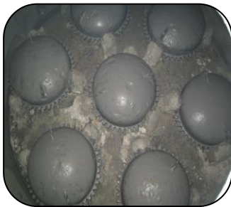
Ammonia Liquor process vessel operating at 100°C resurfaced with 205 Ceramic HT Fluid
