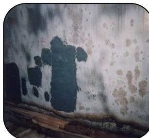
Corroded gas tank holder repaired using 106 Metal Repair Paste XF
