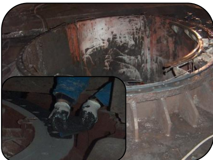
Gasket chocking using 101 Metal Repair Paste
