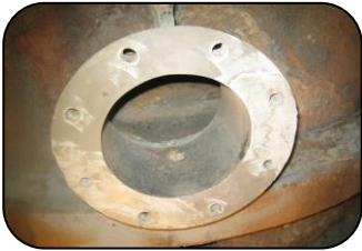
Flange face reforming using 101 Metal Repair Paste
