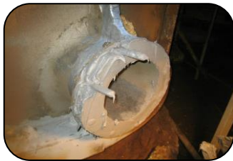
Flange face reforming using 101 Metal Repair Paste
