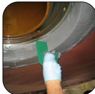
Metal surfaces resurfaced using 101 Metal Repair Paste
